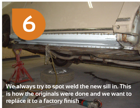
Next step is to cut and fit the inner sill
